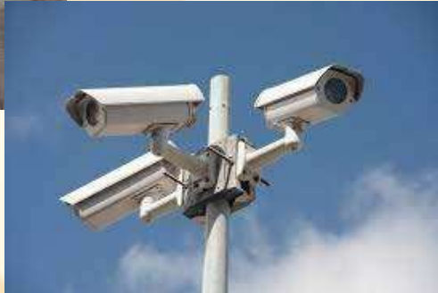
CCTV systems Installa-tion & commissioning
