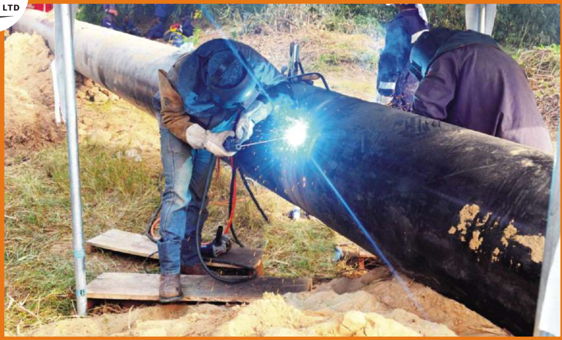
Construction of 36" x 20km Dangote Refinery & Fertiliser Gas Pipeline
