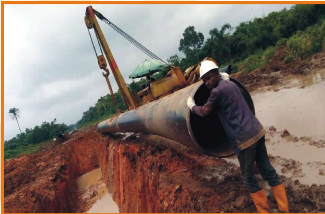
Construction of 36" x 20km Dangote Refinery & Fertiliser Gas Pipeline
