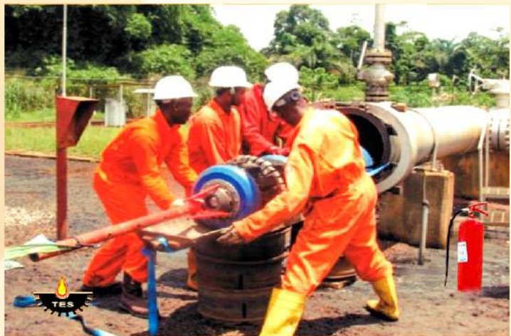
Intelligent Pigging of 18" x 34km Oben-Sapele Gas Pipeline
