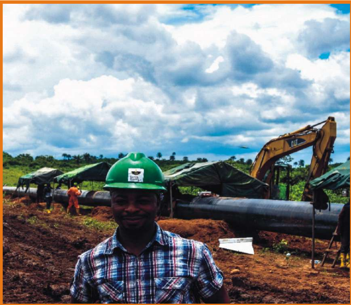
Construction of 36" x 20km Dangote Refinery & Fertiliser Gas Pipeline
