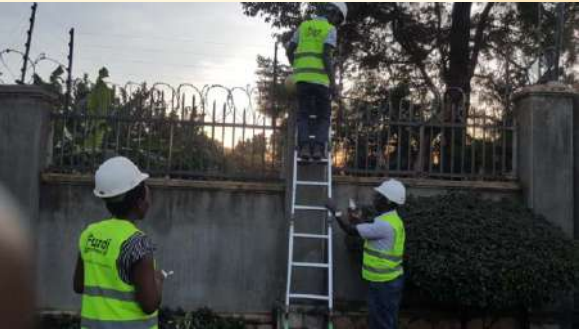
Installation of electric razor fence, CCTV, Lights
