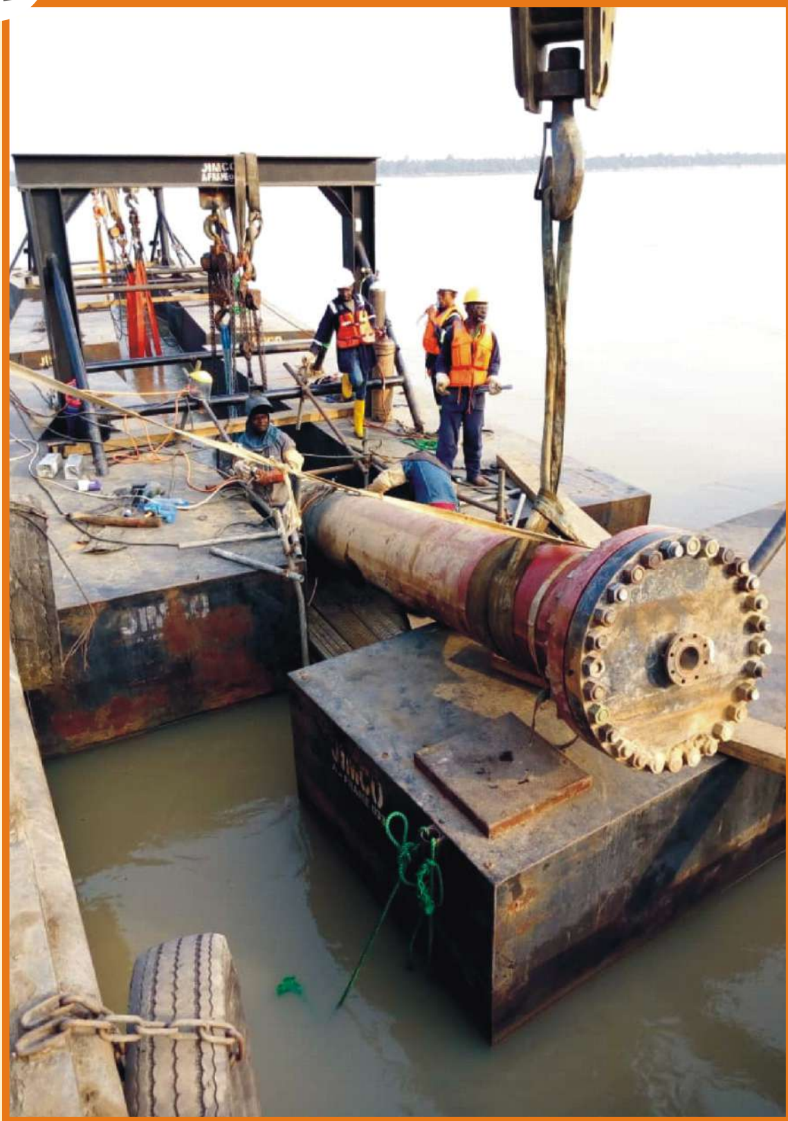
24" x 1.3km River Niger Agip Kwale-Akri Gas Pipeline Repair
